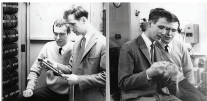
Two photographs of Howard Flack (wearing the suit) and me working on the Ferranti Pegasus Mark II computer. We often had to change the valve (tubes for you Americans!) boards.
